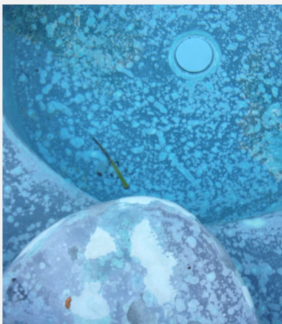
Discoloration seen on an unprotected dark grey plaster spa. Spalling is also seen on the top step.
