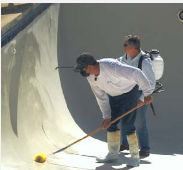
MicroGlass being applied to a newly plastered pool to prevent etching.
