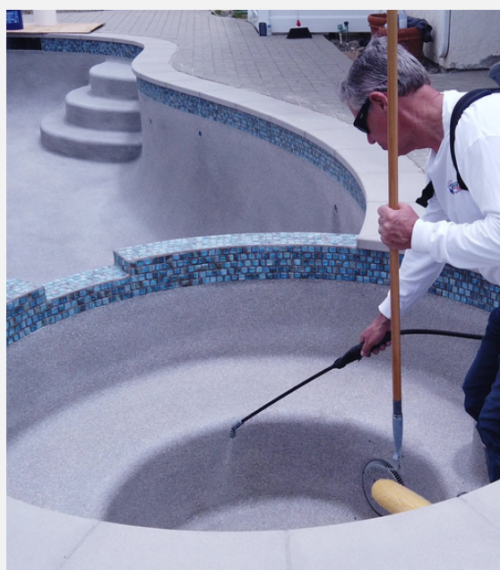
MicroGlass being applied to protect the colored cement paste of an existing pebble pool.
